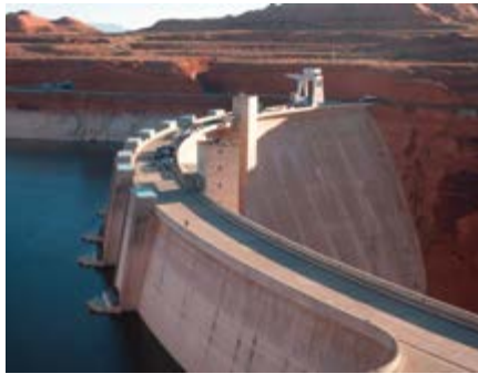
Pumps and pumping stations power supply
